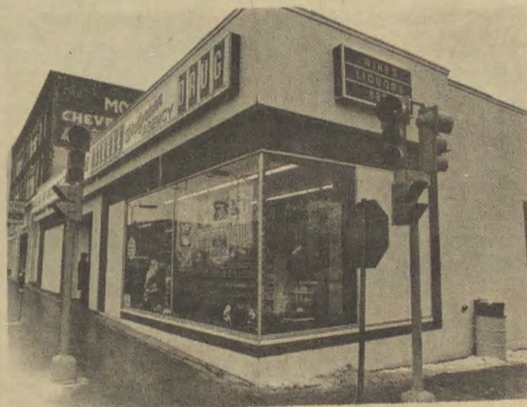
New signal lights installed at the intersection of Maple and Main Streets were turned on this week.
