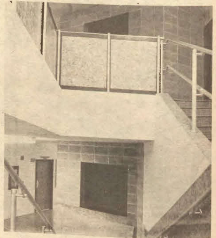
THE BLACK HOLES IN AMES Lab School walls are evidence of elevator construction going on there. Elevators are being constructed in Ames and in Karges Center to accommodate handicapped people. The project, to be completed in November, will cost $144,000. Photo by Al Peterson.
