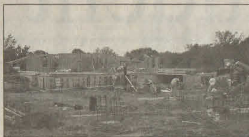
Ground broke on June 28 for the $11.5 million South Fork Suites residence hall. Cost of living on campus has increased over the last three years by $50 to help cover the construction costs. Photo by Teresa Schmitt
