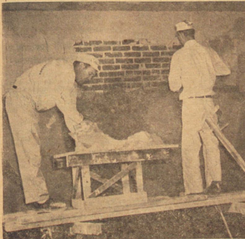
PLASTERERS WORK ON LIBRARY—Two members of a plastering crew apply the primary coat to an interior wall of one room in the soon-to-be-completed Chalmer Davee Library. Despite many delays, the new stone and brick building is expected to be ready for occupancy by spring.
