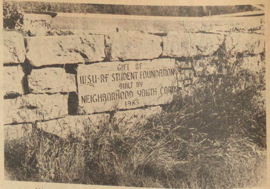
Weeds begin to cover the stonework on the stage.
