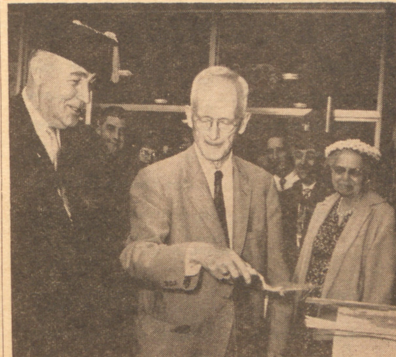
CORNERSTONE CEREMONIES for the new physical education building were highlighted Wednesday when Dr. R. A. Karges smoothed out the last cement for the building which has been named after him. On hand to assist was President of the College E. H. Kleinpell.
