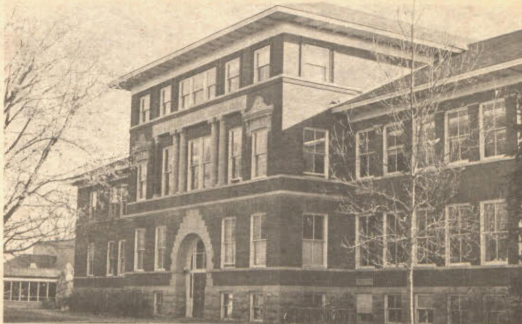
BUDGETED FOR DEMOLITION IN 1978, South Hall may again become a center of controversy on campus. The building has housed every academic
