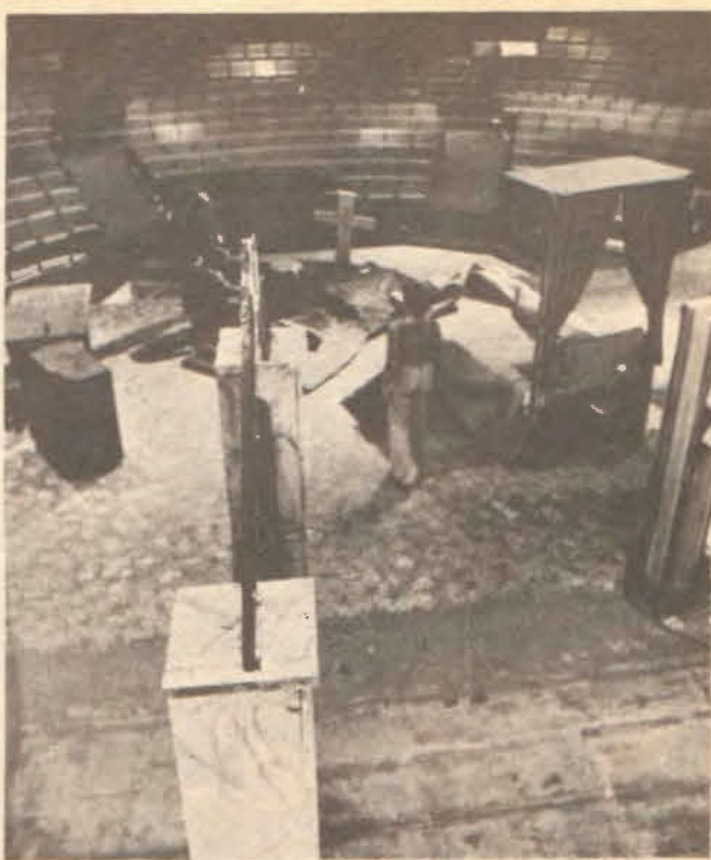
THE SET BEGINS to come to life as the construction nears completion. The night when the seats will be full and the applause grand is long-awaited.
