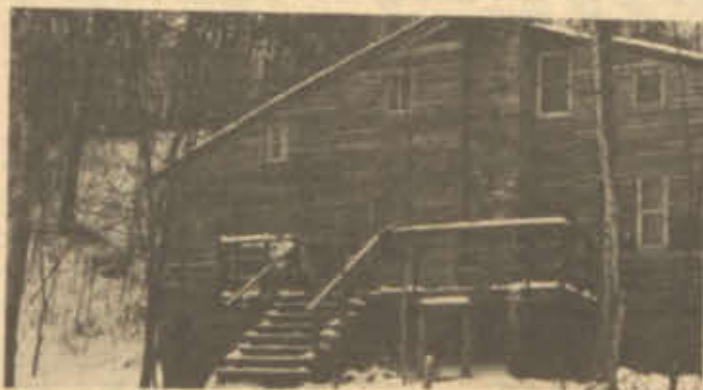
THE CHALET provides living space for some of the 46 people now living in the commune. Photo by Bill McGrath
