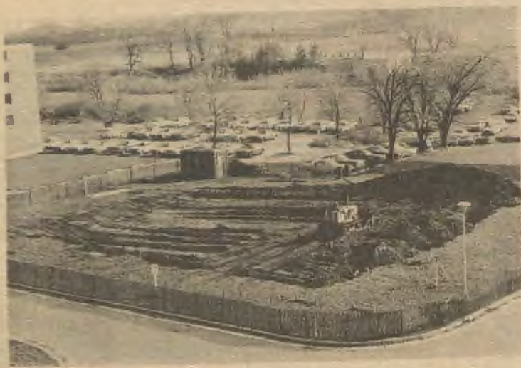
Greenhouse construction starts.
