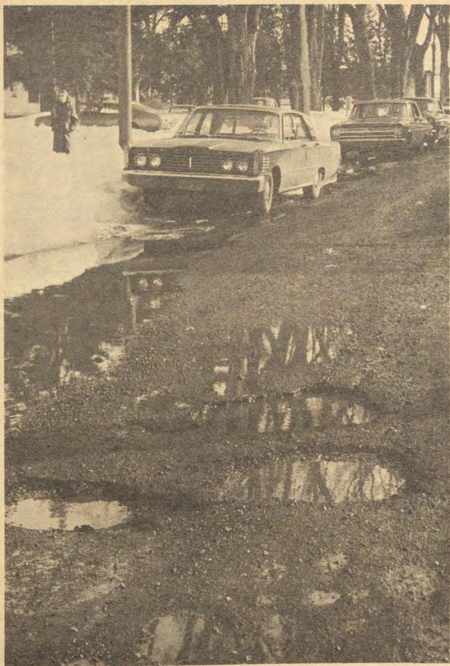
The road by the Davee library is definitely deteriorating in the spring thaw.
