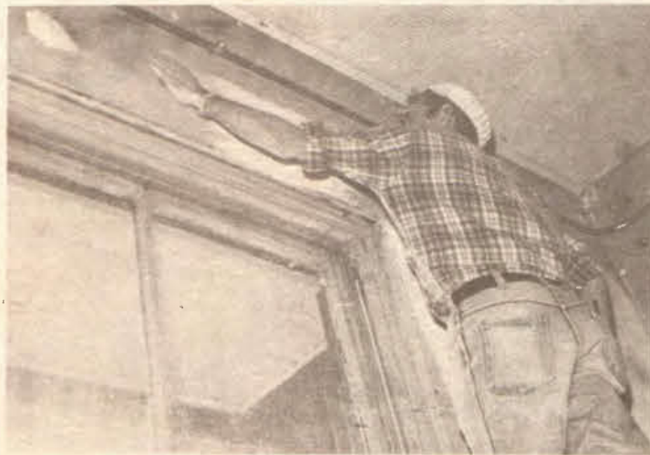
SOUTH HALL is undergoing an internal facelift and preparing for its new inhabitants from Hathorn Hall. Gene Giebler makes some last minute measurements before applying a coat of paint. Photo by Pat Hildebrant.
