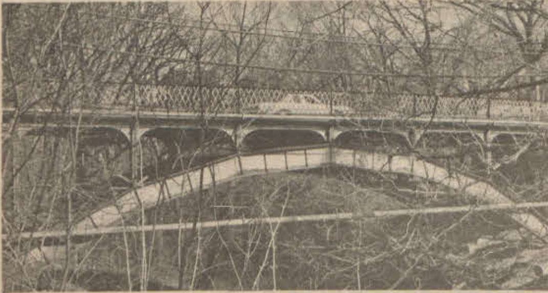
SOUTH MAIN STREET will be rebuilt starting June 1. The June starting time is to avoid student traffic that is present during the school year. Photo by Mary Meysembourg.
