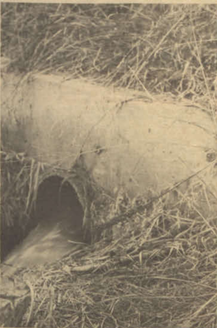
TREATED SEWAGE FLOWS into the Kinnickinnic from the River Falls treatment plant. Photo by Scott Swanson.
