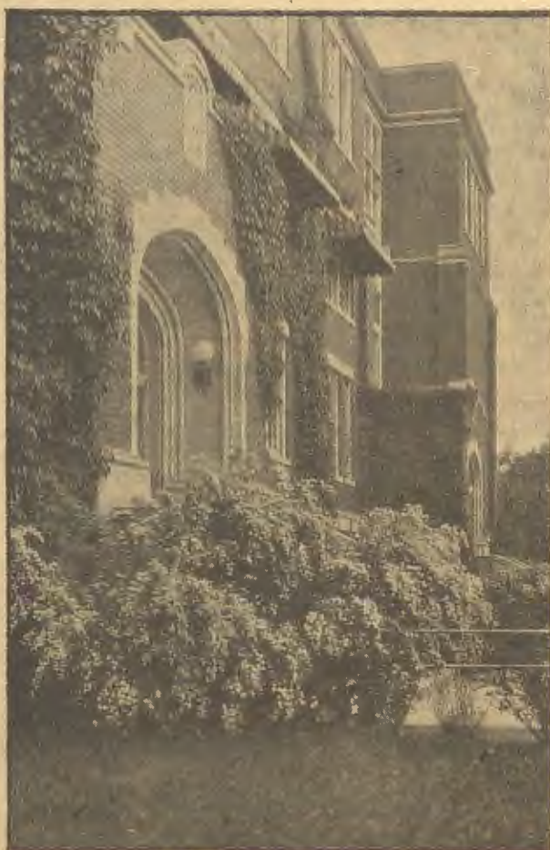
NORTH HALL contains administrative offices, men's gymnasium, the main auditorium, the campus training school, science labs, classrooms, men's lounge, and the swimming pool.
