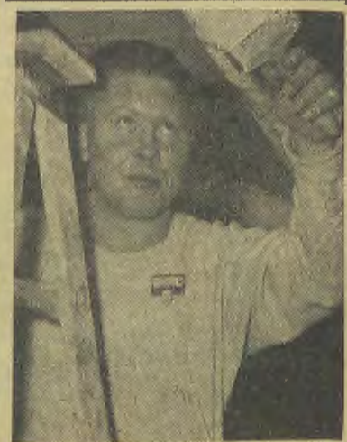
Russ Johannsen, construction worker applies paint to the South Hall lounge.
