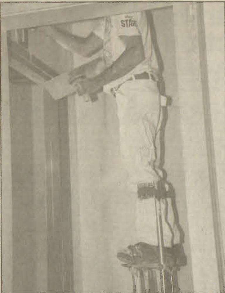
Ryan Brinks / The Student Voice The face of worker Rick Wilbur is hidden as he uses stilts to plaster above the doorways in the second floor of South Hall Wednesday afternoon.
