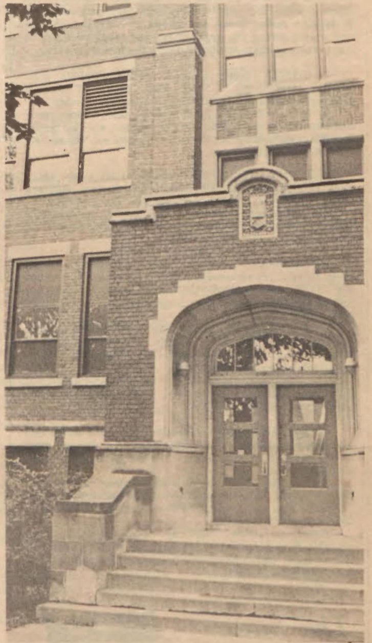
NEW WINDOWS ON THE WORLD are only part of North Hall remodeling project which has escalated in price from $430,000 to $1.5 million. Photo by Doug Reed.
