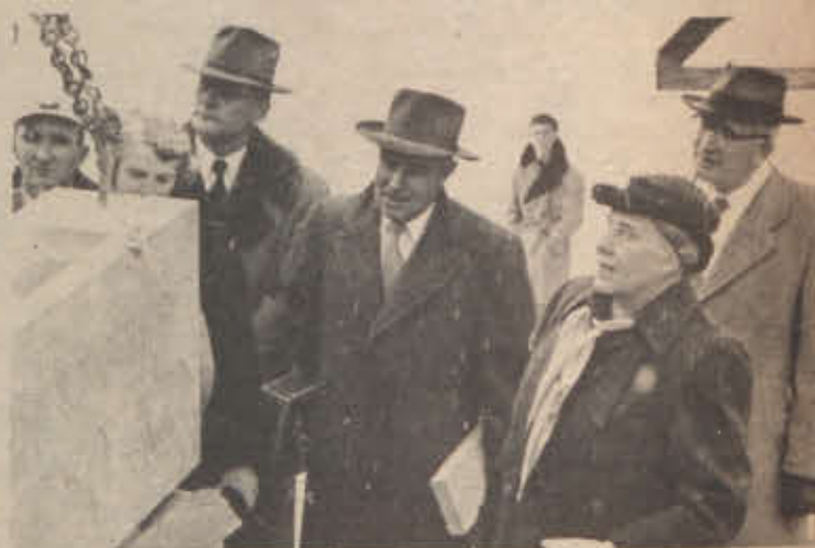
WITH FORMER RIVER FALLS MAYOR AND REGENT H. T. Hagestad, former University President E.H. Kleinpell, Miss Irma Hathorn, and former Regent Chalmer Davee looking on, the cornerstone for Hathorn Hall, named after Miss Hathorn, is laid in January, 1951. Hagestad and Davee both had later buildings on the UW-RF campus named after them, while the Kleinpell Carrillon in North Hall is named after the former President.
