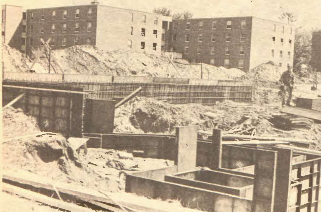
THE FOOTINGS have been laid and the walls are going up on the veterinary medicine clinic scheduled for completion 14 months and one million dollars from now. Photo by Allen Pederson.
