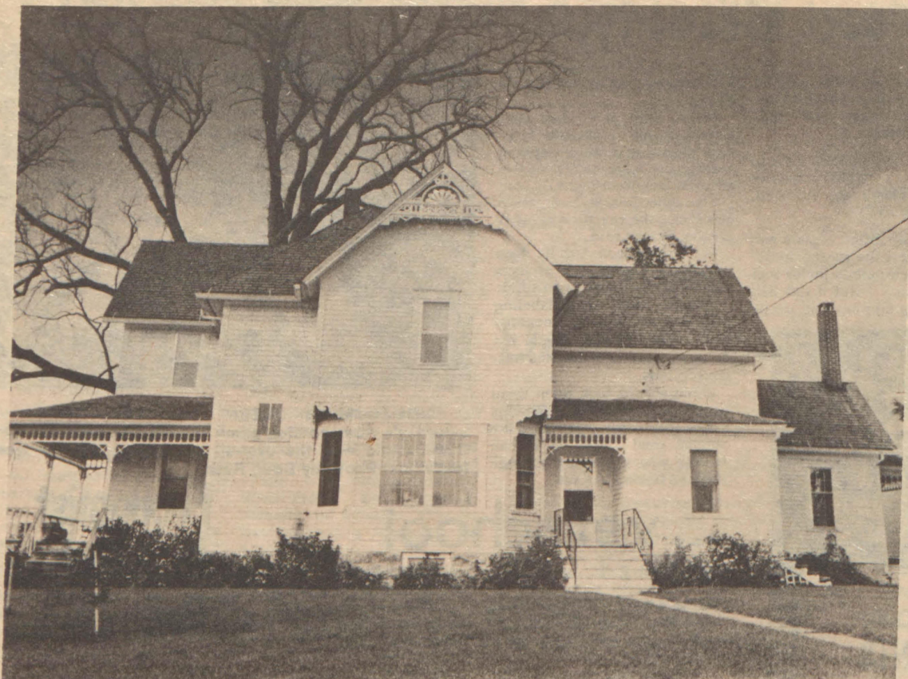
The Wallace Mehlberg home has 21 sides, 10 doors and almost as many porches.
